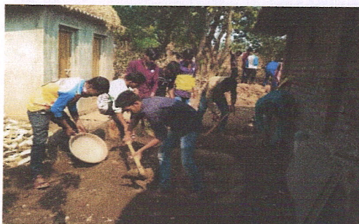
(Soak Pit Construction)
