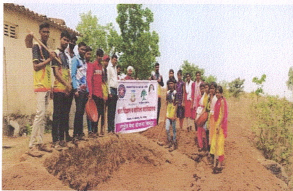
(Compost Pit Construction)
