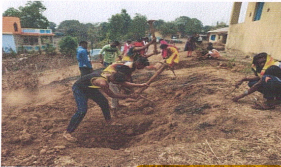
(Soak Pit Construction)
