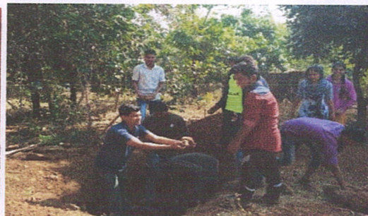
(Soak Pit Construction)
